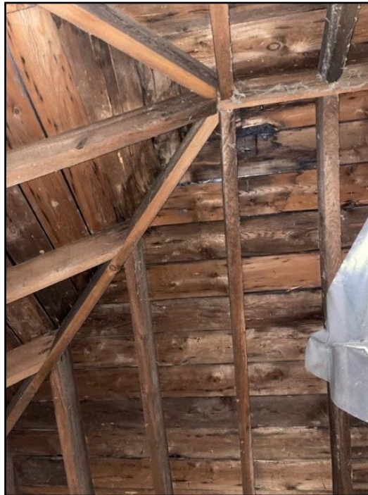
Rafter and Plank sheathing
