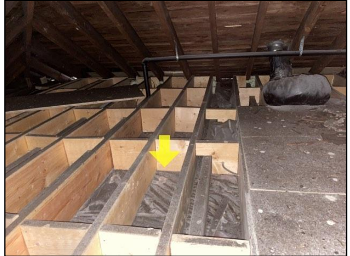
Insulation not yet install
