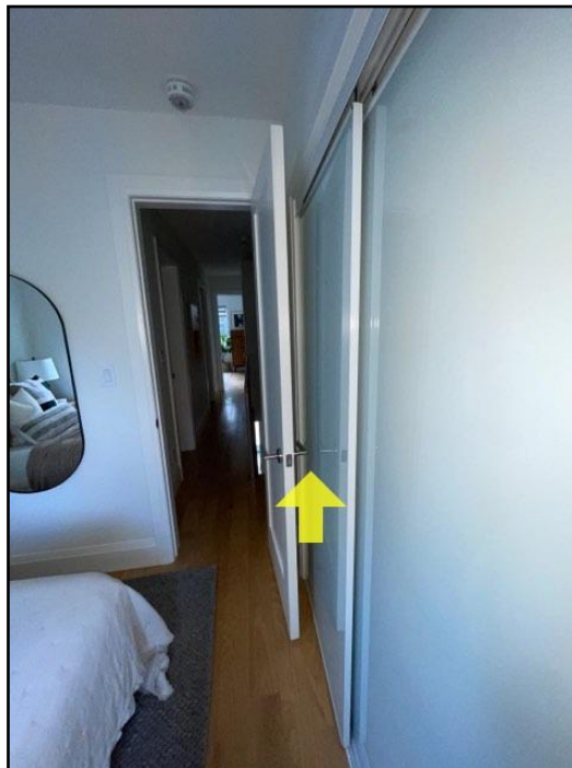
Example : At Second Floor Rear Bedroom
